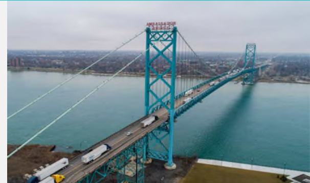
Ambassador Bridge Privately Owned & Operated
